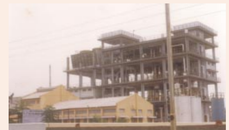
Integrated Pesticide Plant
